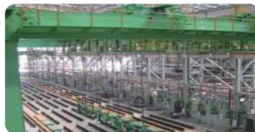
5 WELDING SERVICE GANTRY
