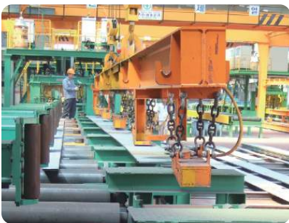
1 SUB-MATERIAL HANDLING CRANE
