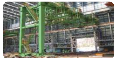
6 WELDING SERVICE GANTRY
